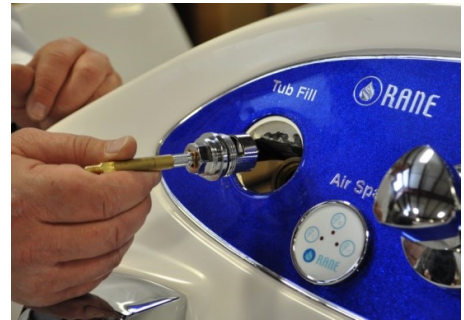
Step 9: Insert and carefully thread in new valve stem. Hand tighten.
