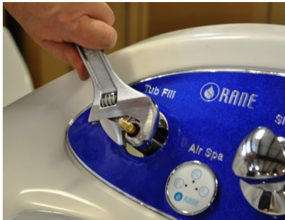
Step 7: Using a crescent wrench, remove part E (fig. 1).
