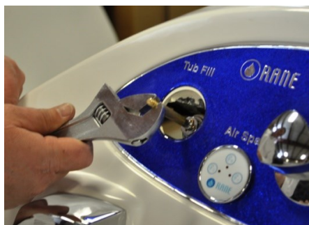
Step 8: Use crescent wrench on square tip of the valve stem and remove.
