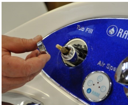
Step 5: Using a crescent wrench, remove part C (fig. 1).
