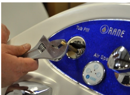
Step 10: Use crescent wrench on square tip of the valve stem and tighten till it stops. Note: Be careful not to over tighten and snap the stem.
